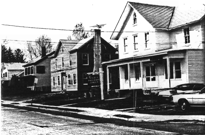
Streetscape: E. side Prospect Ave., N from Church St.
