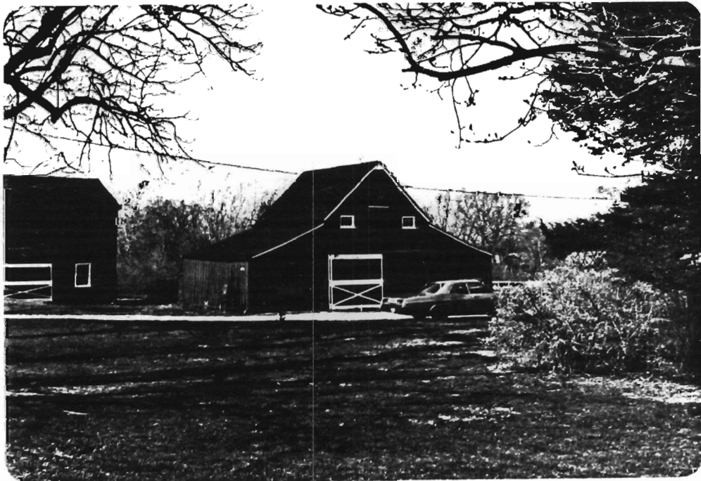
Wagon Shed B, view to NE.
